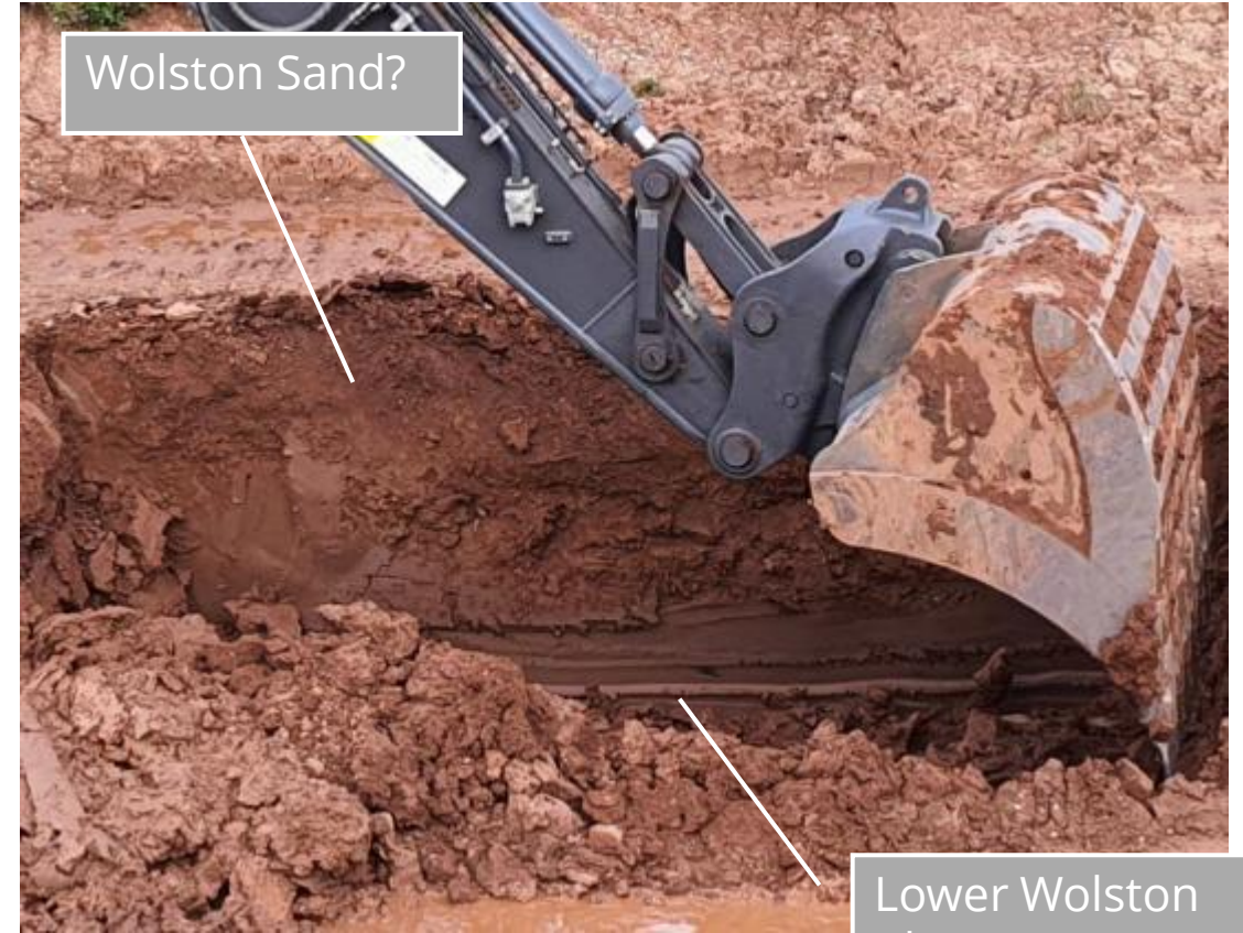
Image - Trial pit in Park Lane Cutting
